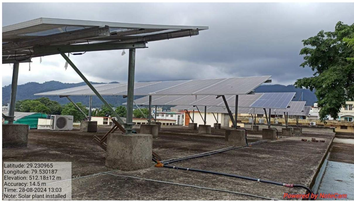
Solar panels with 36 KW capacity have been operationalized, with the electricity generated linked with the national grid.
