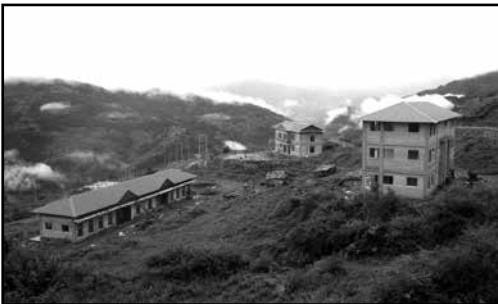
Building of Mountain Training Centre at Garma, Solukhumbu under construction
