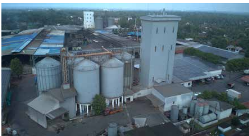
Ekala Feed Milling Facility
